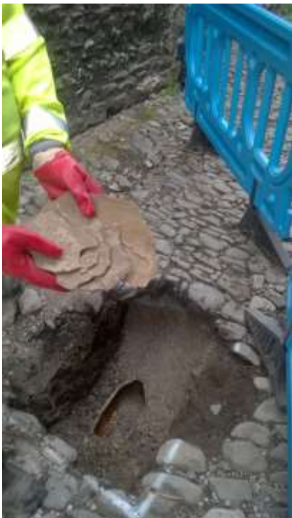
Figure 11 (left): A grout like deposit was found to be lining the inside of the culvert pipes. Figure 12 (right): A gas pipe crossing within the culvert barrel in The Square.
