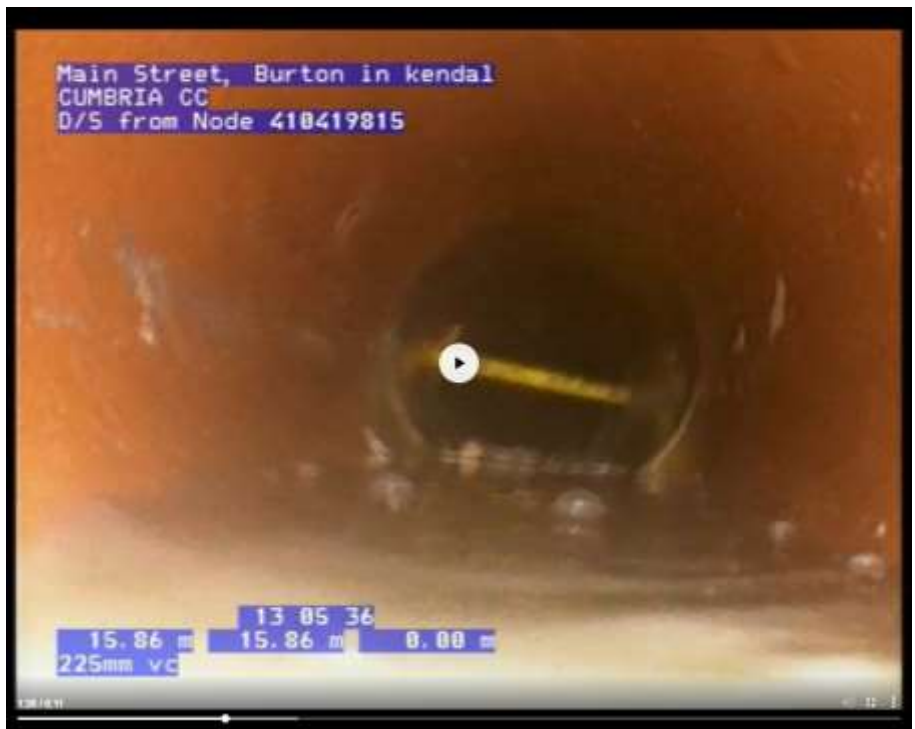
Figure 11 (left): A grout like deposit was found to be lining the inside of the culvert pipes. Figure 12 (right): A gas pipe crossing within the culvert barrel in The Square.
